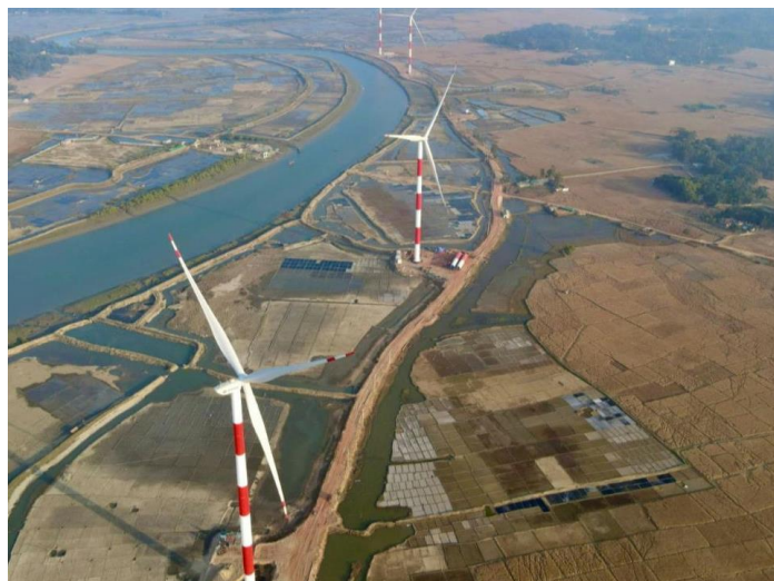
Figure 5: Khurushkul, Cox’s Bazar 60 MW On-Grid Wind Turbine
