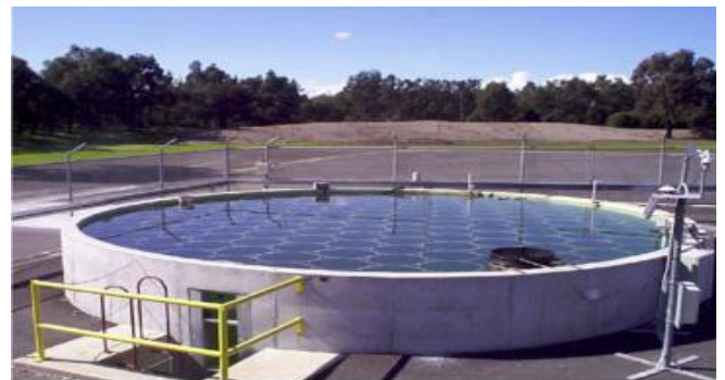
Fig. 3 A 50m 2 experimental salinity gradient solar pond at RMIT University
