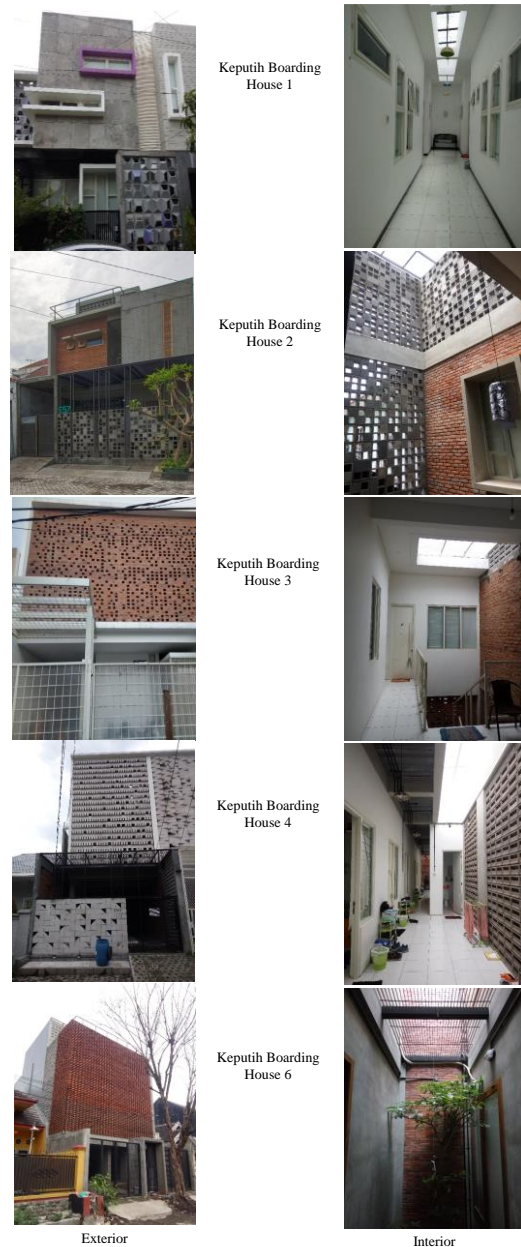
Figure 2: Front exterior and interior view of Keputih boarding house
