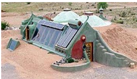
Figure 1: Aerial view of an 'Earthship'. Source: Reynolds, www.dreamgreenhomes
